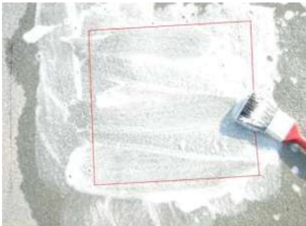
Figure 9. Cleaning of the bituminous membrane.
