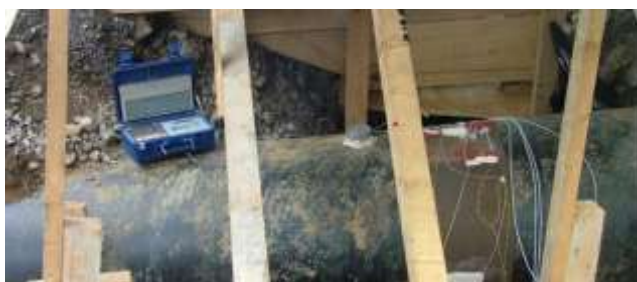
Figure 2. Measurement setup on the oil transmission pipeline [10]
