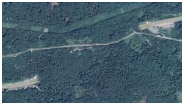
Figure 1. Tunnel “Veliki Gložac” with oil pipeline passing over it
