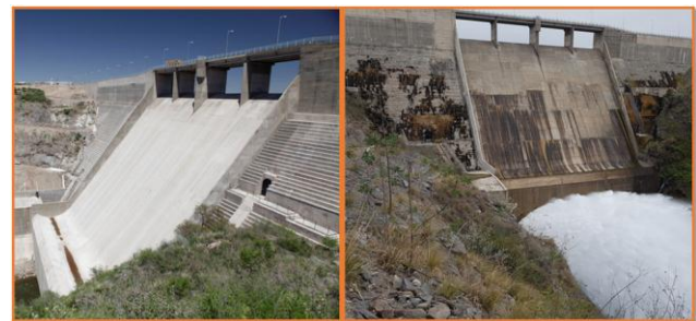
Figure 1. Photos. The dam presents the day of the inauguration, and five years later. There is upwelling of water on the wall waters down by leaks
