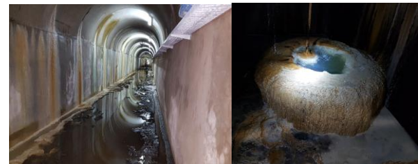
through the body of the dam.
