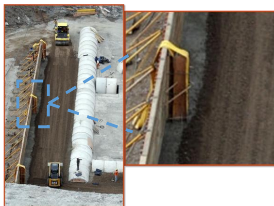
Figure 4. Photos. Shows the lack of detail in the placement of the gasket water-stop.
