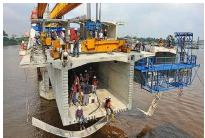
Figure 3.2. Deck cross section and cantilevered techniques construction of Lekki Bridge (Julious Berger Plc, 2013)
