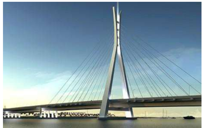
Figure 3.1. Lekki cable stayed bridge (Julious Berger Plc, 2013)
