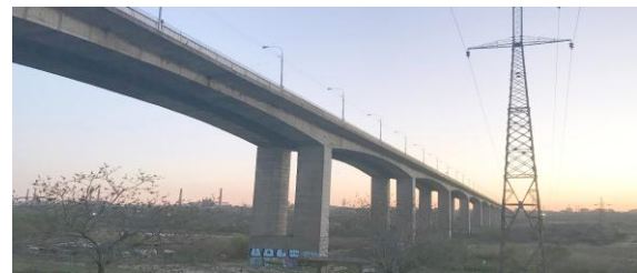
Figure 4. Viaduct – pillar view
