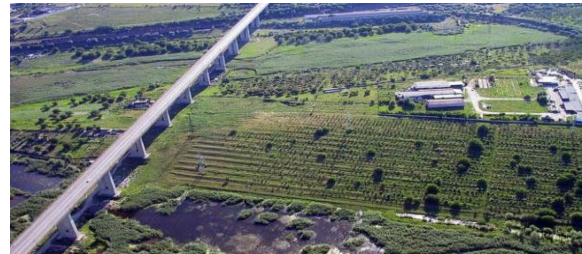
Figure 3. Viaduct – sky view
