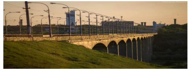
Figure 2. Viaduct – Combinatului Street
