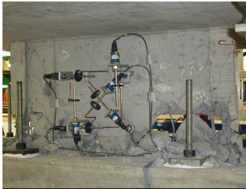
Figure 7(a). Photo of the specimen SC in failure stage (taken at the sixth run PGA=2.0g)
