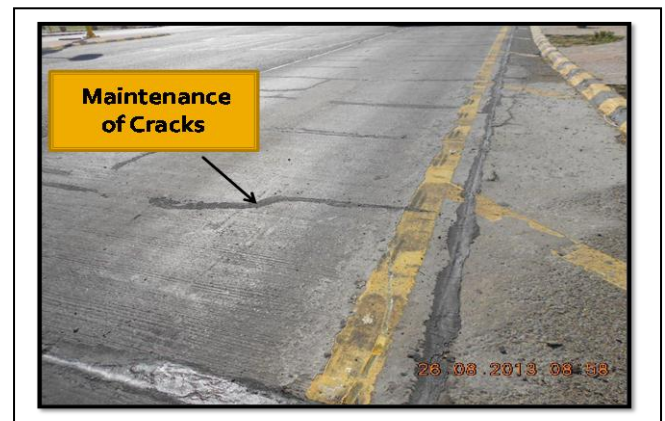
Figure # 8 ; Maintenance of cracks by crack sealing
