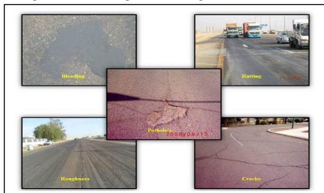
Figure # 1; Deformation of asphalt pavements
