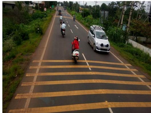
Figure 4 Transverse bar marking for traffic calming
