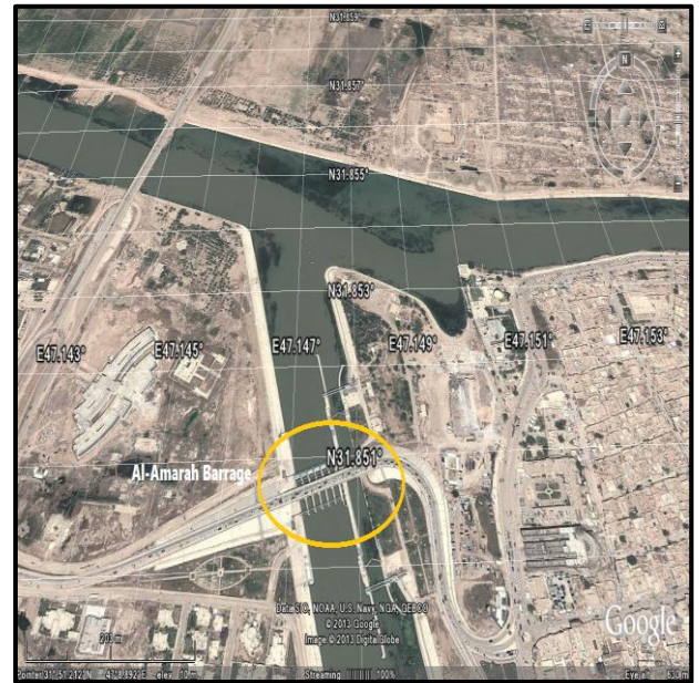
Figure 2. Location of Al-Amarah Barrage [18]
