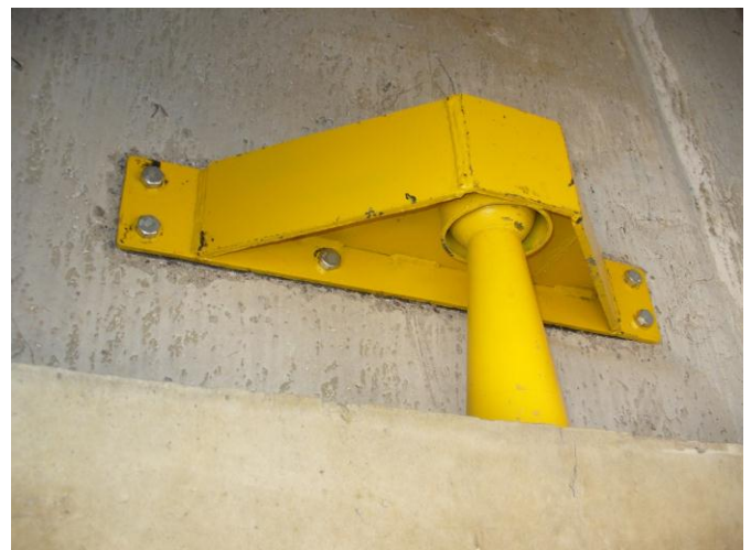
Figure 13. Damper used in the bridge in Sorocayense
