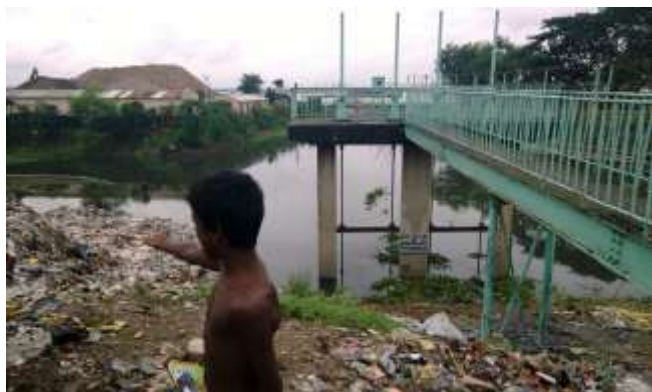
Figure - 4: A boy showing Rayerbazar sluice gate on a canal which flows to Buriganga River with contaminated water.
