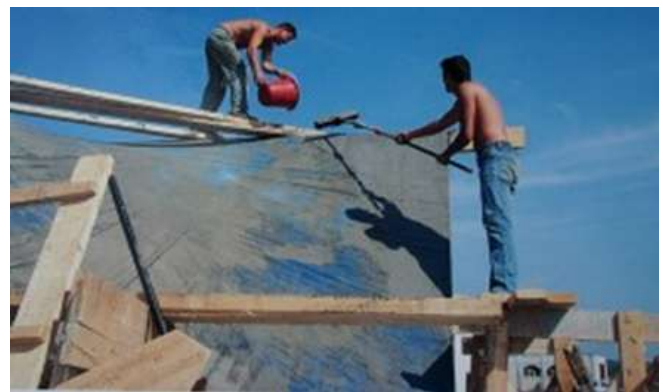
Figure 3. Roof Zed Construction process.
