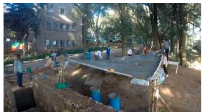
Figure 4. Latex concrete roof made in Ethiopin by the Architecture Institute. ( http://www.hebel.arch.ethz.ch )
