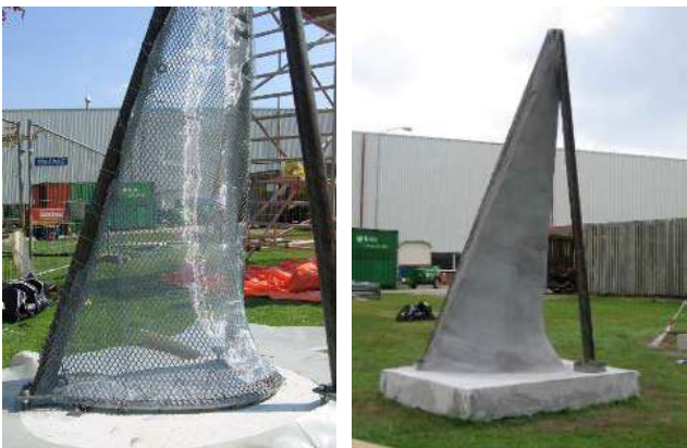
Figure 2. Eindhoven prototype, mesh casted with shotcrete. ( http://www.arnopronk.com/bestanden/PaperArno%20pronk-def%20_3_.pdf )
