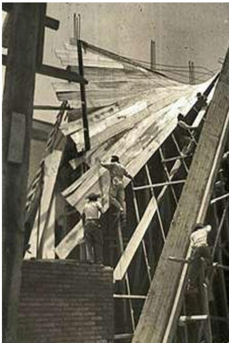
Figure 5. Candela's innovative formwork construction.
