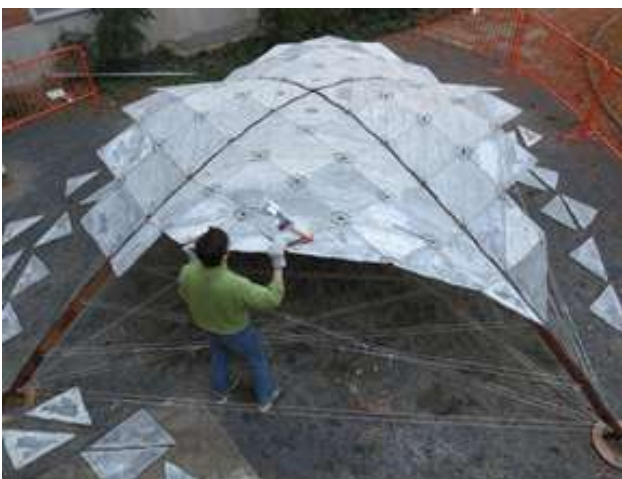
Figure 8. Standart vaults construction. ( http://formfindinglab.princeton.edu/news/realisation-pre-cast-segmented-form-found-shell/attachment/serguei-bagrianski-princeton-concrete-shell/ )
