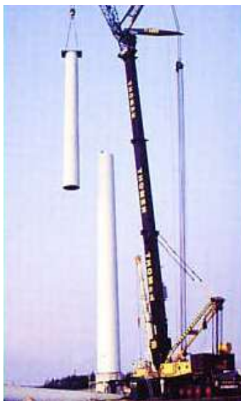
Fig. 4 Nordex N43 tower during construction.
