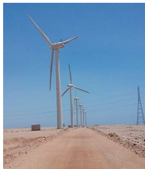
Fig. 1 Nordex wind turbine towers at Zafarana wind farm.
