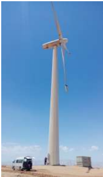
Fig. 3 Typical Nordex N43 wind turbine tower at Zafarana wind farm.
