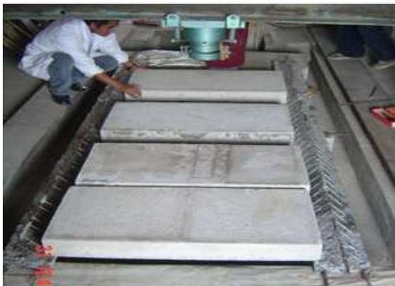
Figure 12. Roof's construction using prefabricated beams
