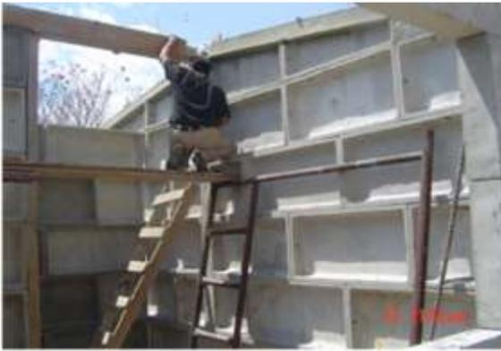
Figure 11. Ensemble of walls using prefabricated elements
