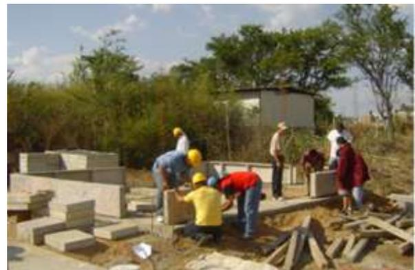
Figure 10. Placement and leveling of prefabricated elements
