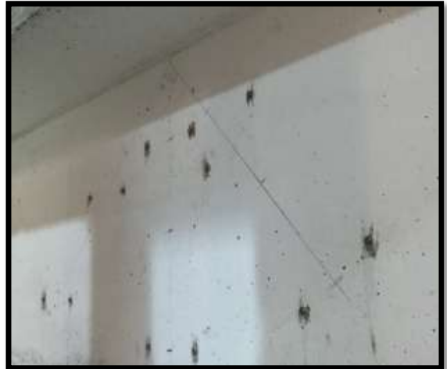
Figure (4) strain points to measure the concrete strain
