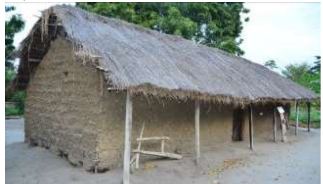
Figure 2. A Kwere e Doe-Bantu house - Nyumba Ya Wakwere Wadoe. Communities resides in Coastal Regions of Bagamoyo and Kibaha districts
