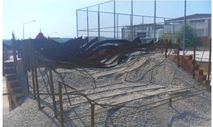
Fig. 3. Placement of the fill material in the lake
