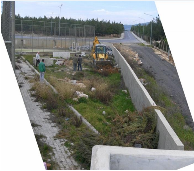
Fig. 2. The initial sight of the construction area.
