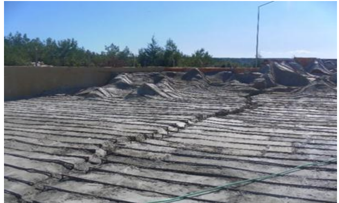
Fig. 4. Formation of the concrete surfaces
