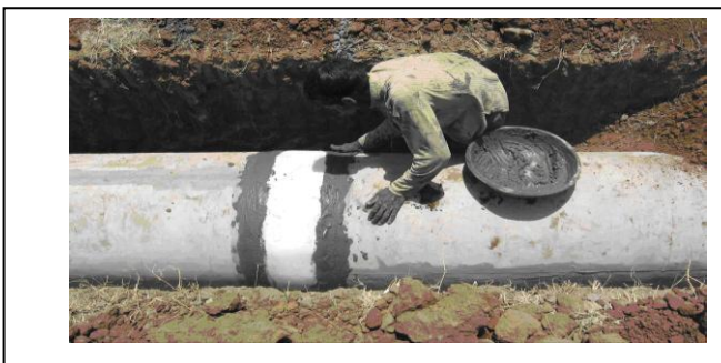
Figure 2. RCC pipes connected using geosynthetic joint
