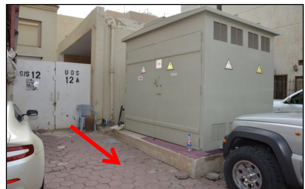
Fig. 4. Qortuba substation no. 12 indicating highest magnetic field levels
