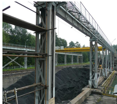
Fig. 7. View of the crane
