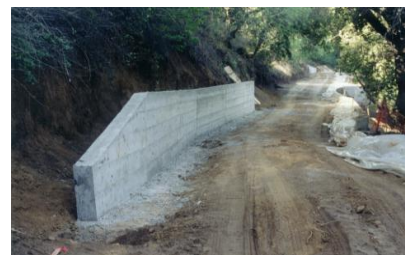
Figure 7. Concrete wall barrier.
