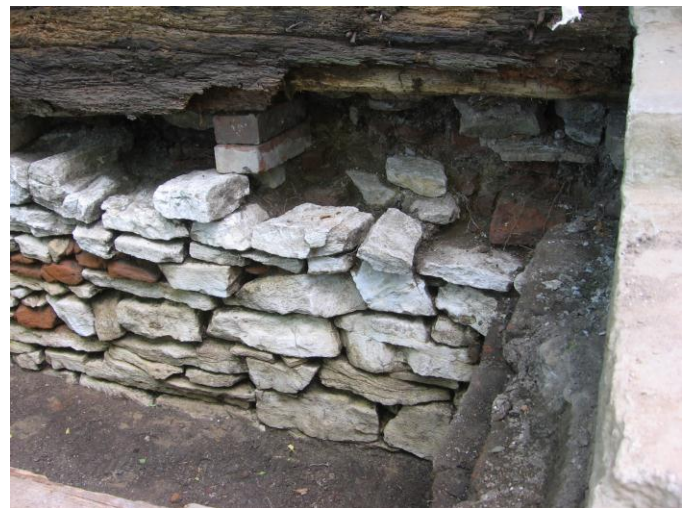
Figure 2. Appearance of the exposed foundation walls of different construction.
