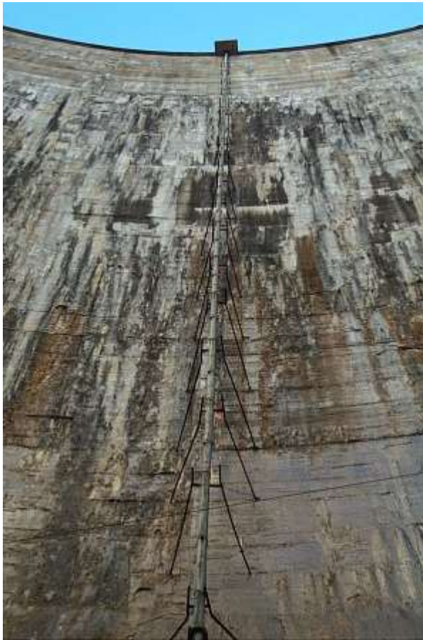
Figure 2. Pendulum in La Cohilla Dam.
