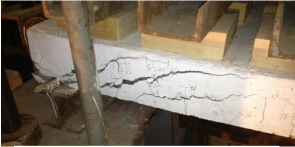
Figure(7): Shear failure of slab S1.
