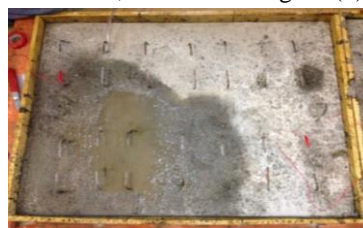
Figure (1a): Pre-slab before casting the second layer.
