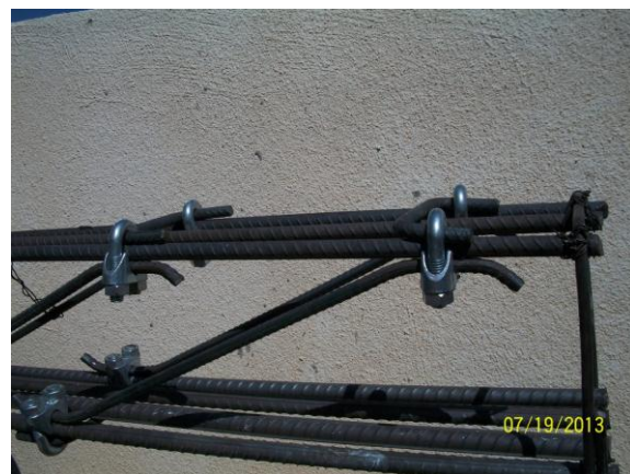
Fig. 2: Typical U-Link swimmer bars
