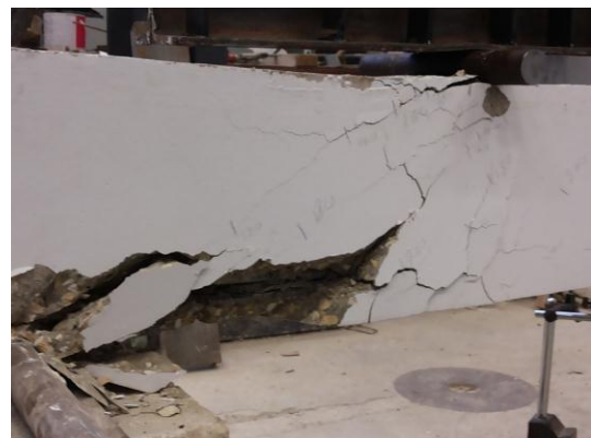
Fig. 5: Beam SSB at failure stage.
