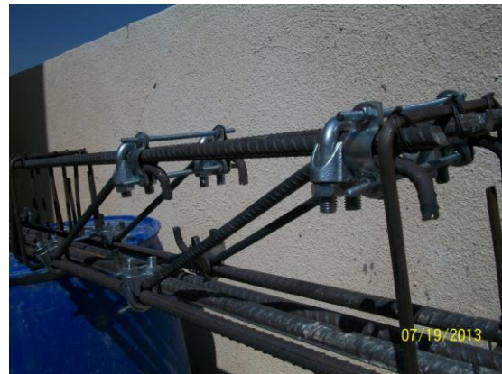
Fig. 1: Typical bolted swimmer bars
