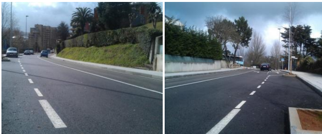
Figure 15. Road in use
