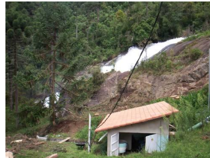
Figure 1: Waterfall and power house
