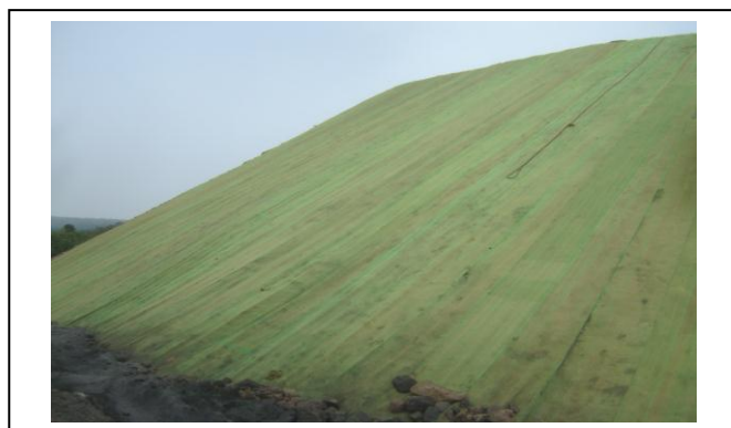
Fig.2. View of the slope of waste dump after covering with soil and blanketing with coir-mat.
