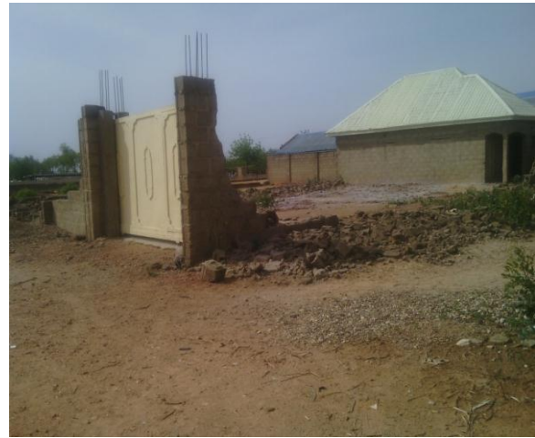
Plate 5: Collapsed block wall fence around Residential Building
