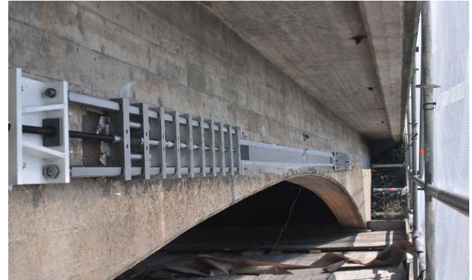
Figure 6. Strengthening of The Nossan bridge in Sweden with two laminates, pre-stressing force of 100 kN in each laminate.
