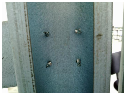
Figure 13. Screw tilting (BC4)
