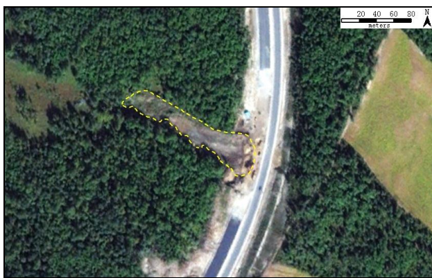
Figure 11. The October 2010 landslide area (Google image)
