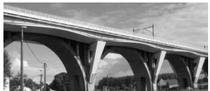
Figure 2. Front view of the new steel super structure
