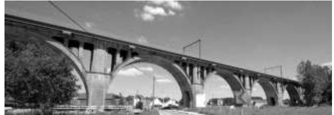
Figure 1. Front view of the historic Pede viaduct.
