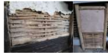
(b) Panel plastered with mud and lime
