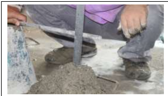
Figurer 2 Slump test
