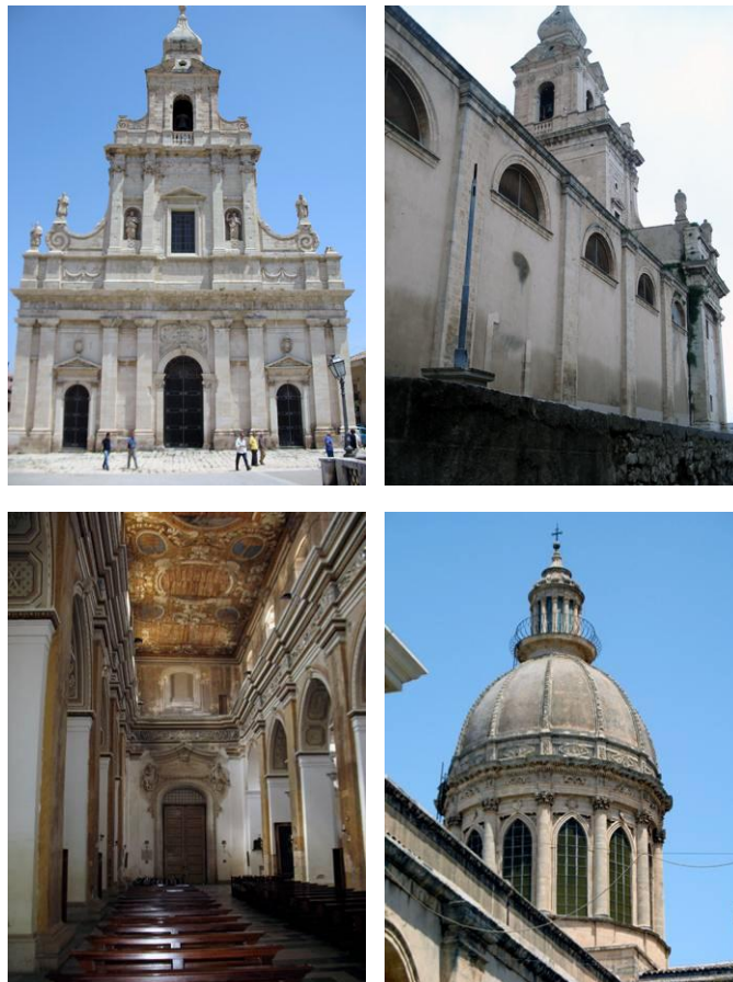
Figures 1-4. Comiso (Ragusa, Sicily), Santa Maria delle Stelle Church, external ed internal views.
