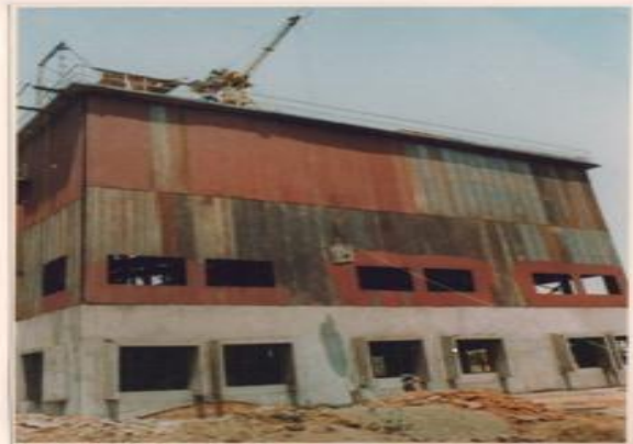
FIG.07 : MINI CLIMBING CRANE HOISTING LOAD WHILE STANDING ON THE ROOF OF THIRD STOREY.
