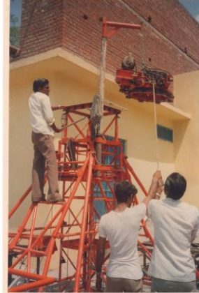
FIG.05 MINNI CLIMBING CRANE UNDER ERECTION. THE ASSEMBLY OF RING GEAR AND PLATFORM CHASIS (WEIGHING ABOUT 170 Kg.) IS BEING LIFTED UP WITH THE HELP OF PIVOTED POLE HOISTING GADGET.
