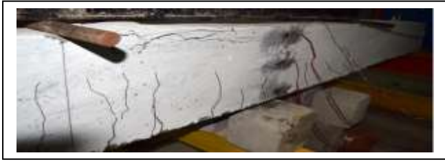
Figure 5. Crushing of concrete in UBPTR specimen
