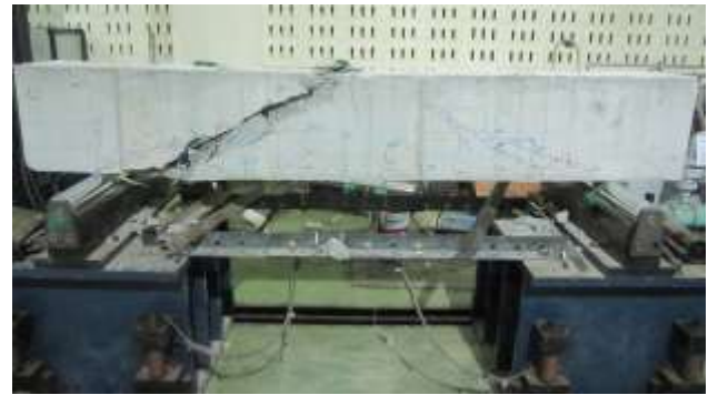
Figure 5. Shear compression failure
