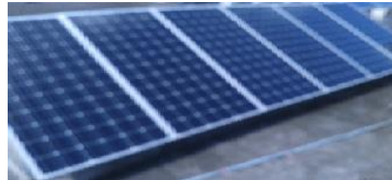
Figure 6. 1.2 kW p PV array at rooftop
