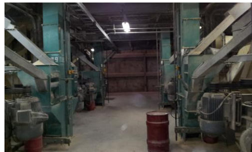
Figure 8. The environment around the equipment installing area
